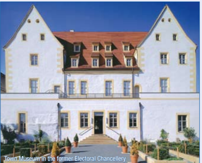
Town Museum in the former Electoral Chancellery
